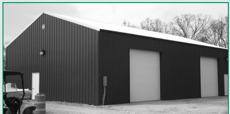
The new maintenance shop
