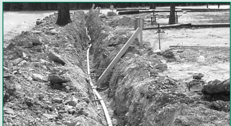
Electrical Upgrade Underway
